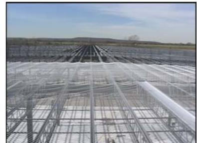
Once construction is complete, the mesh remains as a permanent part of the roof system, providing support for the insulation materials. The product's white color blends well with most fiberglass insulation facings, maintaining an attractive and nearly invisible appearance.
