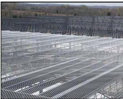
over the secondary roof members, workers can work at the leading edge of the roofing process without being tied off. This freedom from being tied off
