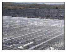
over the secondary roof members, workers can work at the leading edge of the roofing process without being tied off. This freedom from being tied off
