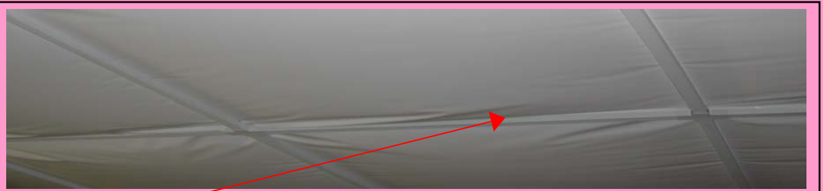
Facing Tabs are secured into White Extrusions while pulling facing tight.
