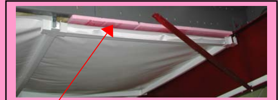
Thermal Blocks installed if required.
